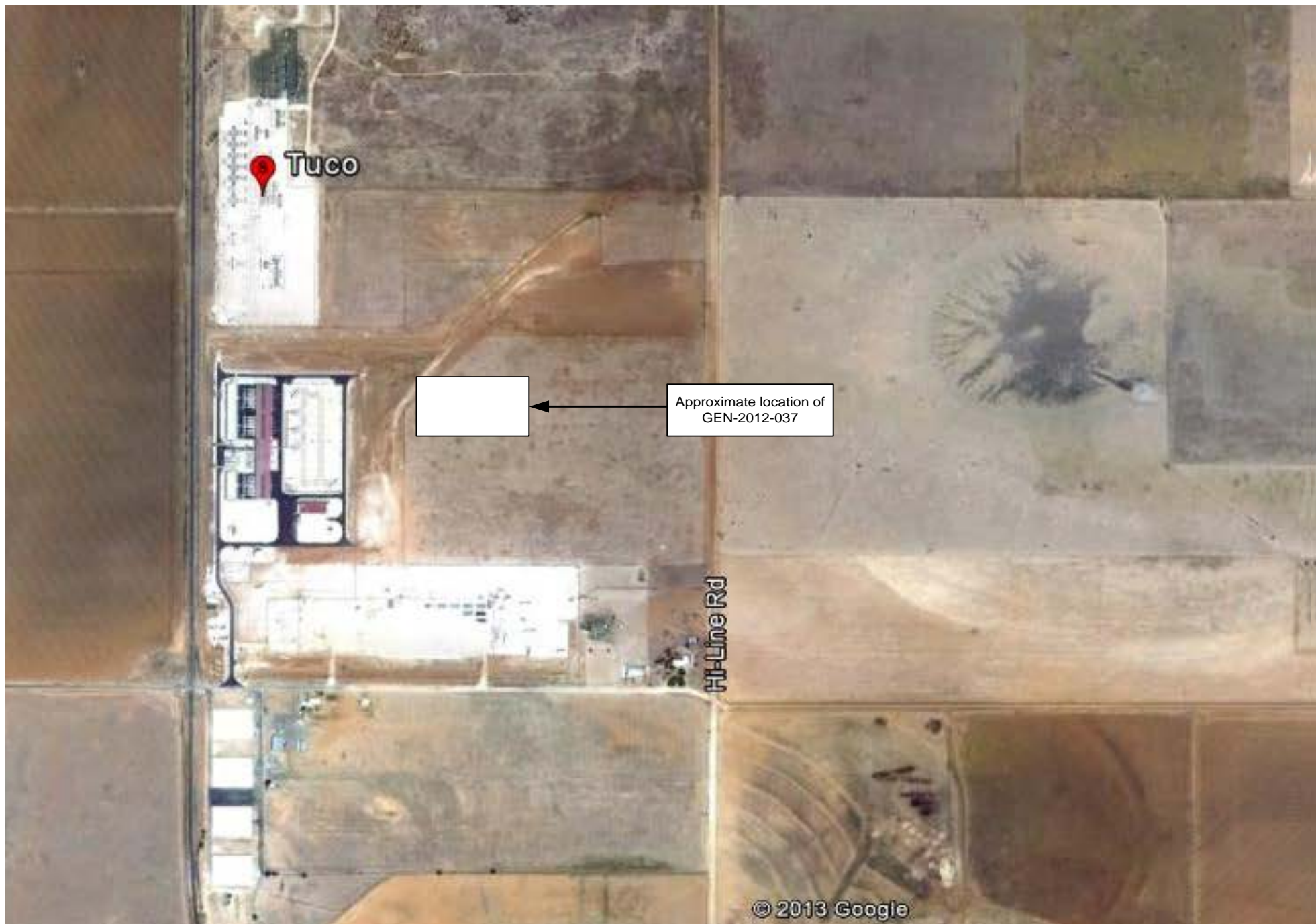
Figure A- 1 Approximate location of proposed Interconnection Customer Combustion Turbine Generator
